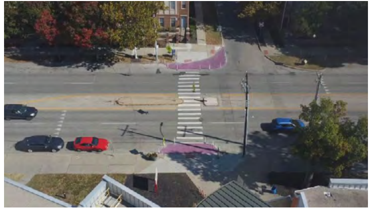
Purple thermoplastic fills curb extensions in Cincinnati. Source: Christian Hauser
