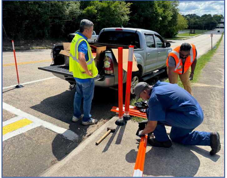
Preparing delineators for installation. Source: Macon-Bibb County.
