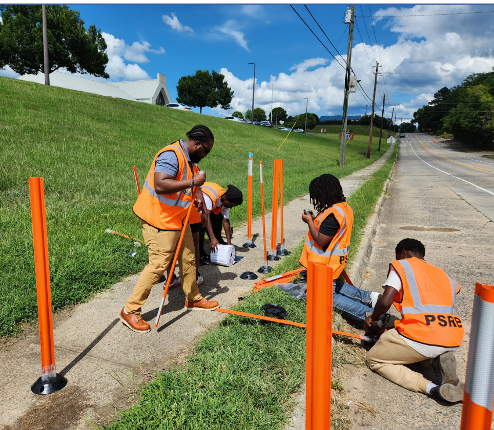
Preparing delineators for installation. Source: Charise Stephens
