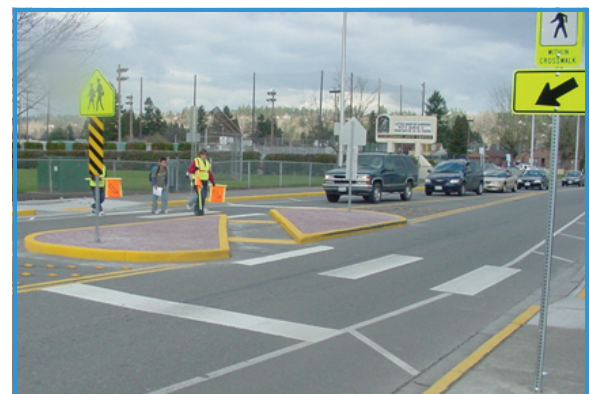
Pedestrian Crossing at Washington Elementary School
